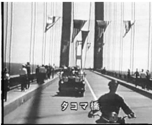
Collapse of Tacoma Bridge (1940, USA)
