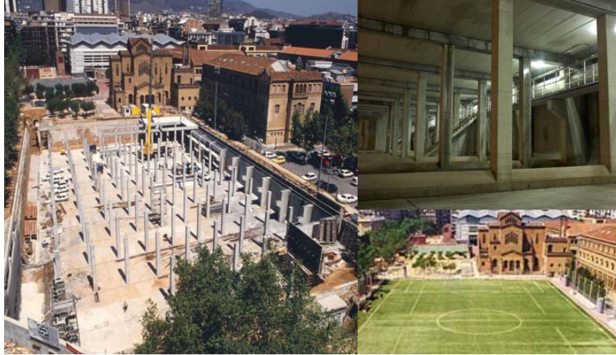
Fig. 10. Retention tank located at Escola Industrial de Barcelona
