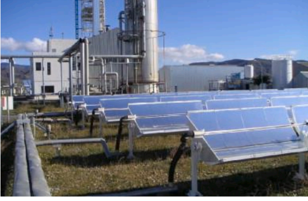
Fig. 3. ACUREX collector loops.
